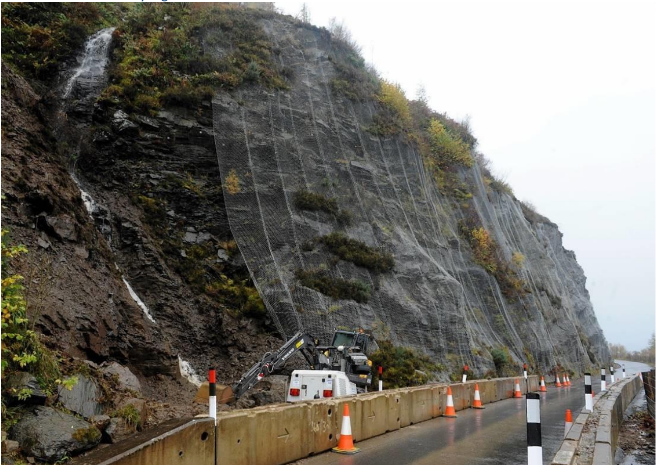
The road is closed every night for work to stabilize the rockface.
